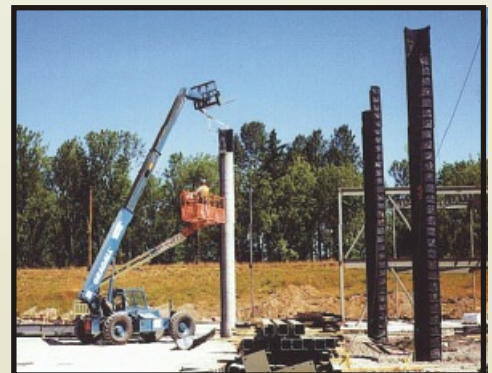
PCF COLUMNS STACKED
