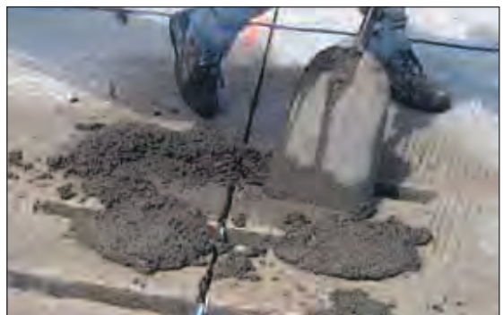
Backfilling the slots with DB Retrofit Mortar.
