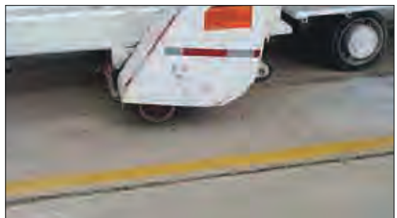
Diamond grinding of pavement lane.
