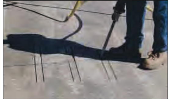
Preparing the slots.
